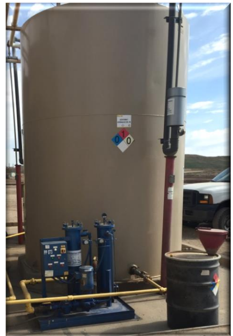
Kidney-Loop Filtration On Bulk Lube Oil Tank
